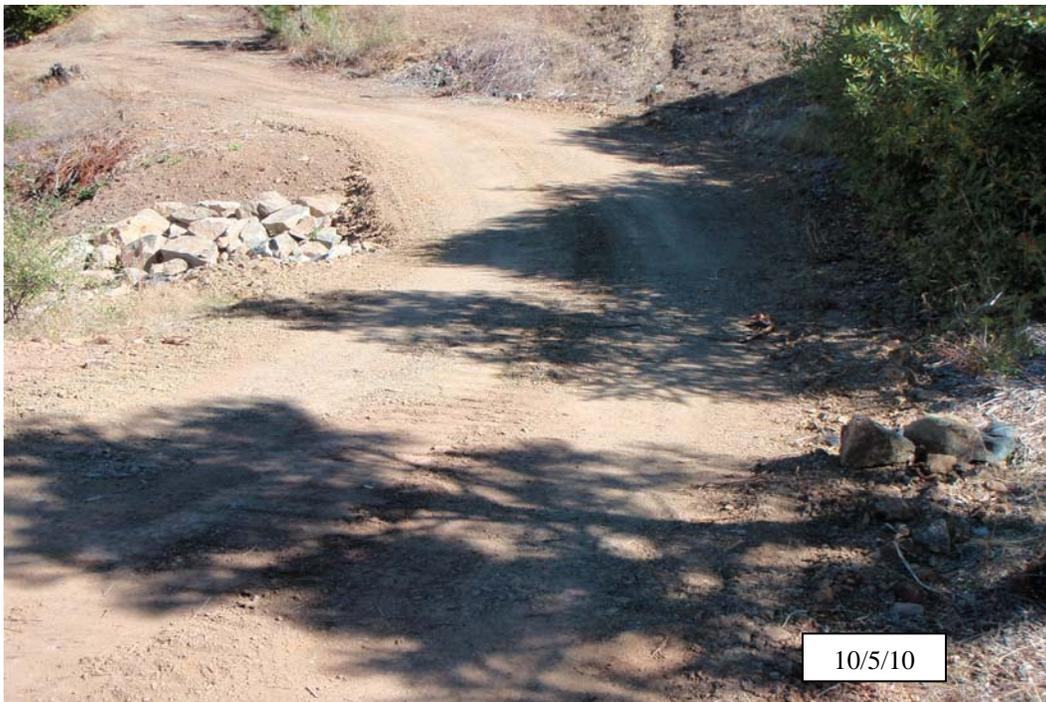
**Photo 10b.** Godfrey/Harris Ranch, site #31, similar view as above, after implementation. View from the left cutbank, looking downstream across the road prism. An armored fill was constructed by dipping the road and armoring the outboard fillslope.
