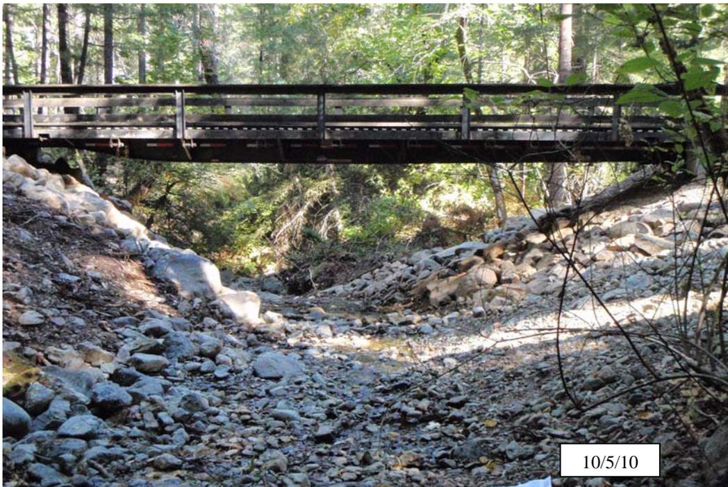
**Photo 7b.** Finley Camp Road #2, site #36, similar view as above, after implementation. View from the TOP of the crossing, looking downstream at the new bridge. The original sideslopes were exhumed and 40yds<sup>3</sup> of 2-3' diameter rock armor was placed on each side to protect the banks from scour and erosion.
