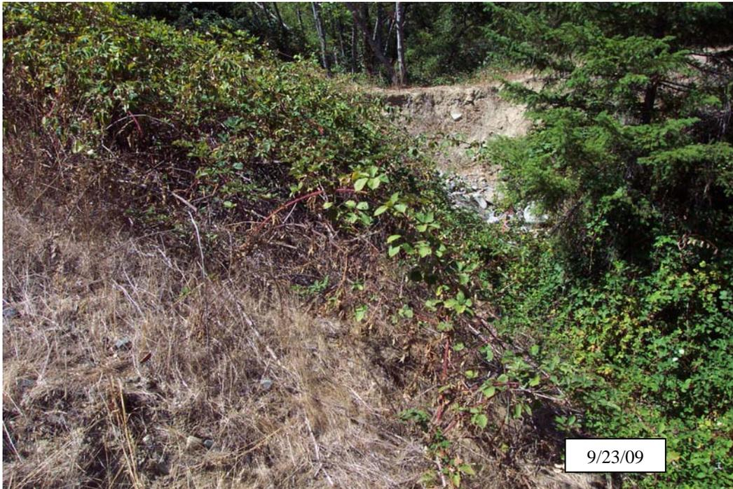
**Photo 1a.** Bloomer Mine Spur #1 Road, site #3, before implementation. View from the bottom of the site, looking upstream at the crossing of a Class II stream. Prior to treatment, there was no drainage structure at this site and the fill was actively eroding.
