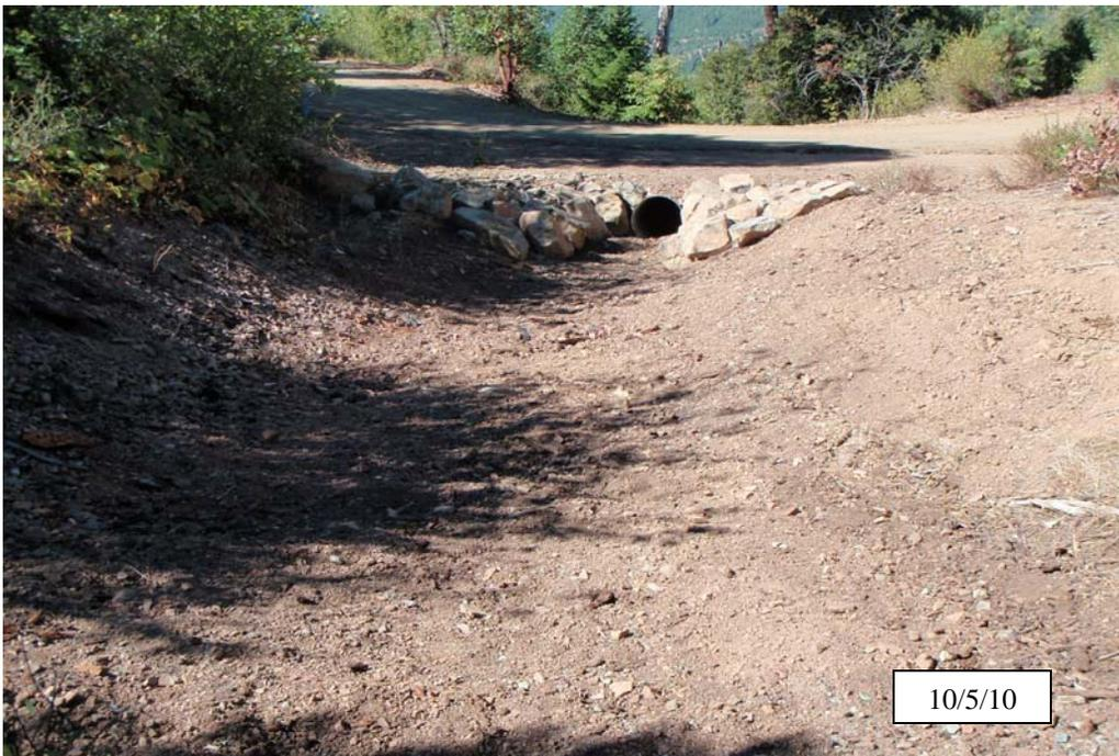
**Photo 9b.** Godfrey/Harris Ranch, site #30, similar view as above, after implementation. View from TOP of the crossing, looking downstream at the new culvert inlet. The channel has been excavated with 2:1 side slopes above the crossing, and a 24 in. diameter  $\times$  80 ft long culvert installed. Rock armor has been placed at the inlet and outlet for fillslope protection.
