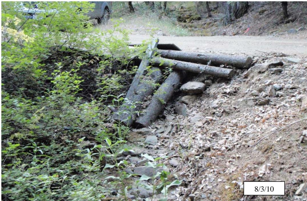
**Photo 3a.** Cecilville/Taylor Road #1, site #42, before implementation. View from the bottom of the site, looking upstream at a crossing of a Class III stream. Prior to treatment, there were two, mostly plugged culverts at this site and a plywood/debris supported outboard fillslope.
