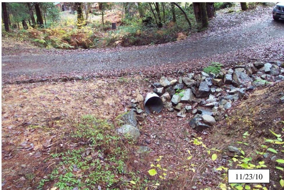
**Photo 11a.** Butler Flat, site #102, similar view as above, after implementation. View from TOP of the crossing, looking downstream at the new culvert inlet. The channel has been excavated with 2:1 side slopes above the crossing, and a 24 in. diameter  $\times$  30 ft long culvert installed. Rock armor has been placed along the right approach, lead-in inboard ditch to minimize future scour from an active spring.
